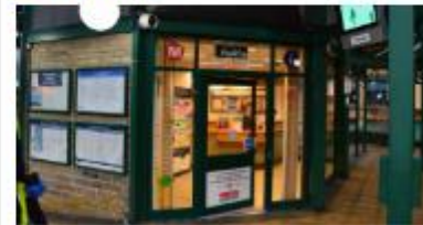
Existing Halifax bus station travel centre, separated from passenger concourse
